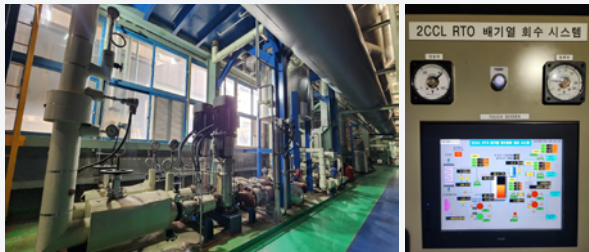
2CCL Exhaust Heat Recovery System (SeAH Coated Metal)
