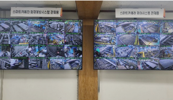
Smart Camera Monitoring (SeAH Steel)
