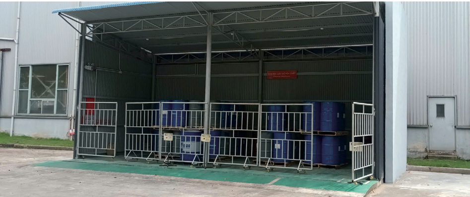
Renovation and New Construction of Chemical Warehouses (SeAH Steel Vina)
