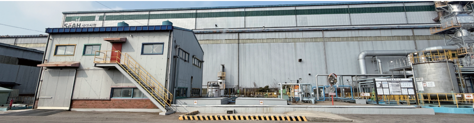
Industrial Water Purification Facility (SeAH Coated Metal)
