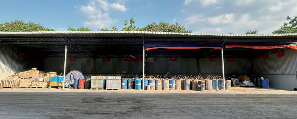
New Construction at the Bien Hoa Plant (SeAH Steel Vina)
